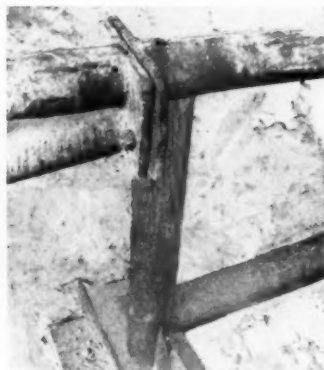
CONNECTORS. —Two similar plates facing each other as braces connect each section, as above.
